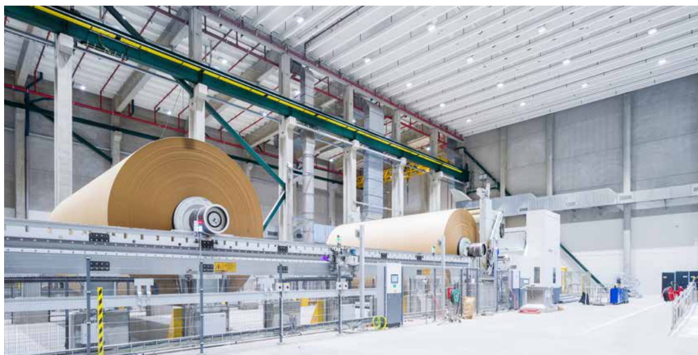
Production at the Obbola paper mill, one of Europe's most modern plants, will increase from the previous 450,000 tonnes of kraftliner to 725,000 tonnes per year.
