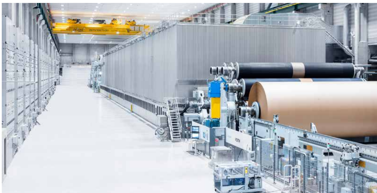
The paper machine in Obbola marks a leap forward in technology in terms of production and process control.
