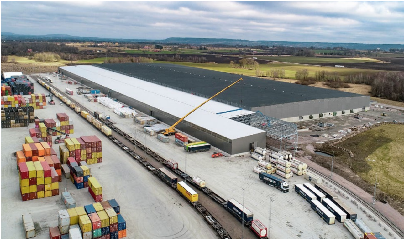
The terminal has a green building rating and is equipped with solar panels. Forklifts running on green electricity handle SCA Logistics' cargoes.
