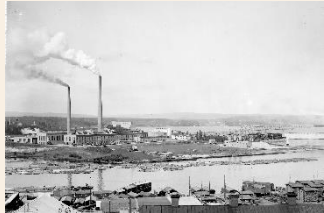
SCA invested in new kraft pulp production with the construction of the Östrand pulp mill
