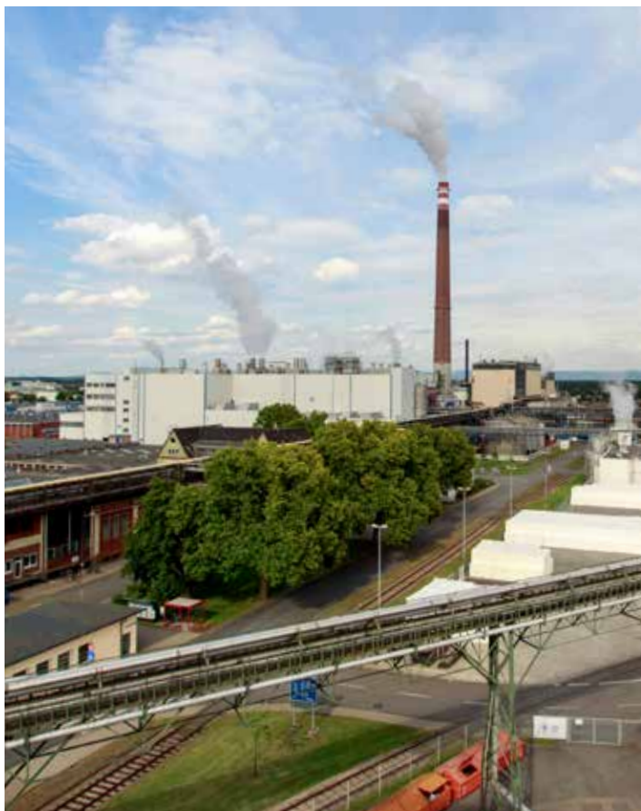
SCA's upgrade of the biogas plant in Mannheim will reduce carbon emissions and increase production efficiency.
